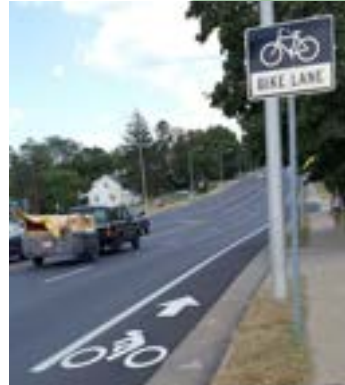
Bike lane signs complement pavement markings.
