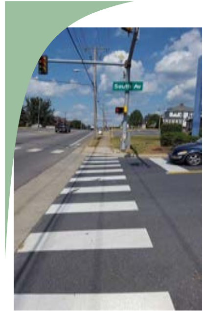
Continental style crosswalk with Pedestrian Signal.
