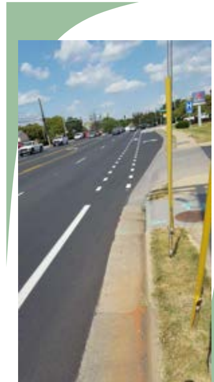
Sidewalk and Bicycle Lane.
