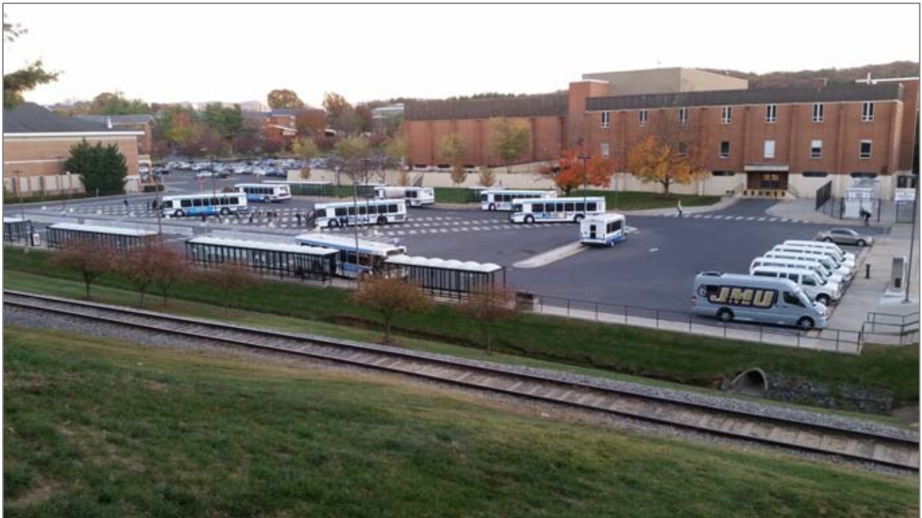
Figure 1-12: Godwin Transit Center
