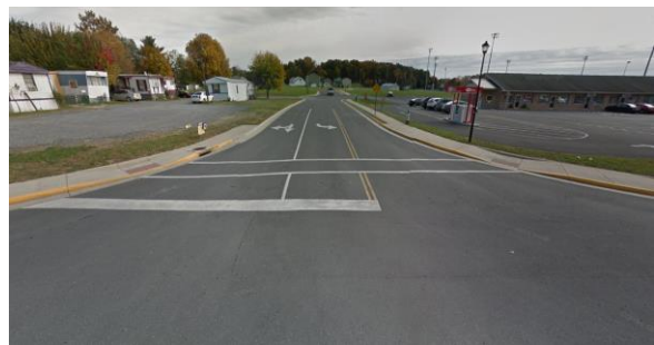
Figure 6: Crosswalk at Dylan Circle with marked crosswalk behind the stop bar
