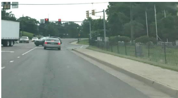
Figure 5: Sidewalk approaching Oakwood Drive northbound with no buffer
