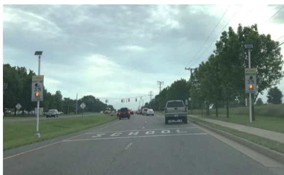
Figure 3: Divided Highway segment of Main Street Approaching School Zone
