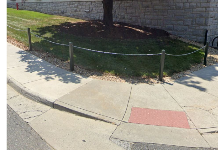
Figure 2 – Wood Post/Chain Fencing
