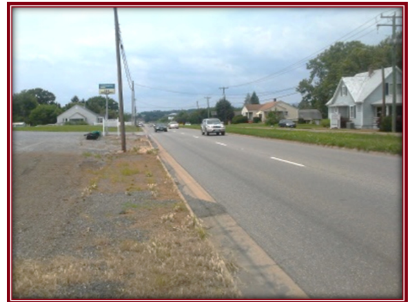
John Wayland Highway looking West towards Garbers Church Road
